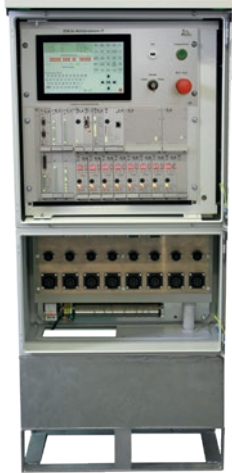
EPB 24 Master for max. 8 power cards or with no power cards*
