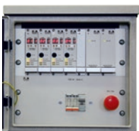
EPB 24 Slave as mast distribution unit for max. 4 power cards
