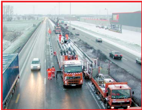
Beginning of the works: Cold, snow
