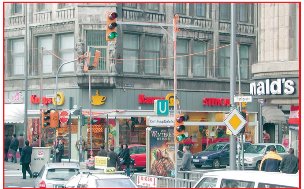
Tallness building site in Cologne: equipment with intersection control device EPB 48 multiprocessor
