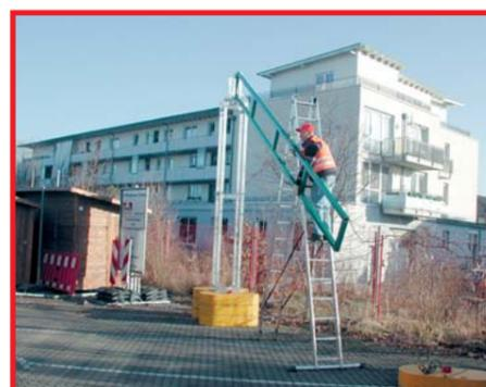
It is hardly believable: Just one person can build up this horizontal mast with a way through height of 4,50 meters and a discharge of 6 meters. This is the great advantage of the use of aluminum.
