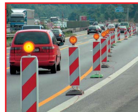
Temporary traffic control light system
