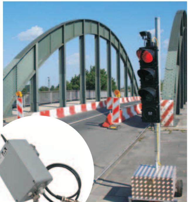
Live information from the road works: the SMS monitoring system sends an SMS, fax or e-mail to the service technician in good time before the batteries have to be changed and when any other faults occur
