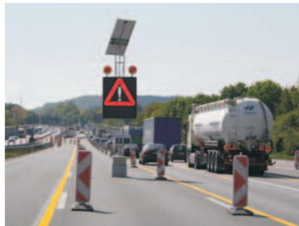
LED alternating traffic signs by MIS GmbH at a hazard point in the roadworks on the A2 motorway at Bielefelder Berg.
