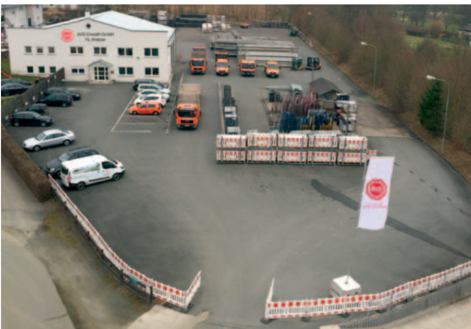
Helicopter view of the new company premises for the AVS Wetzlar branch in Leun an der Lahn, in the state of Hesse
